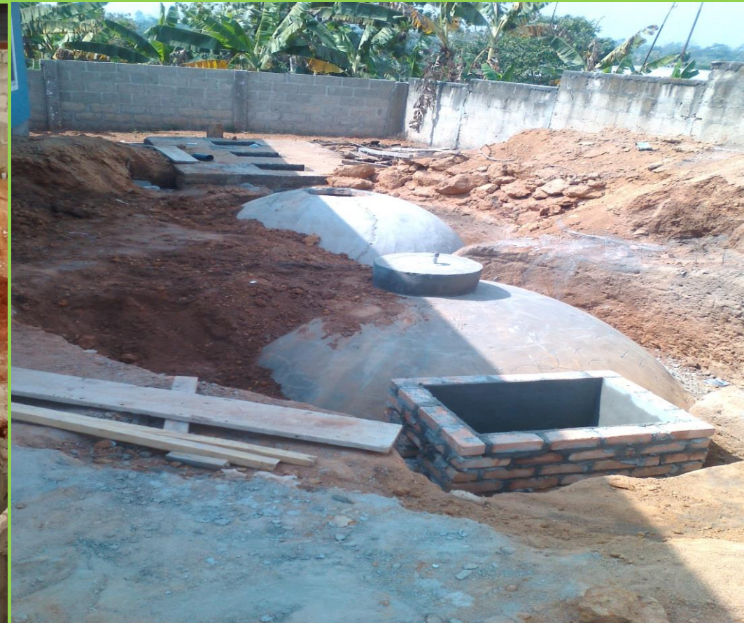
FULL WASTE TREATMENT SYSTEM AT A PRIVATE RESIDENCE IN JUABEN-A-R, TO TREAT THEIR KITCHEN AND TOILET WASTE
