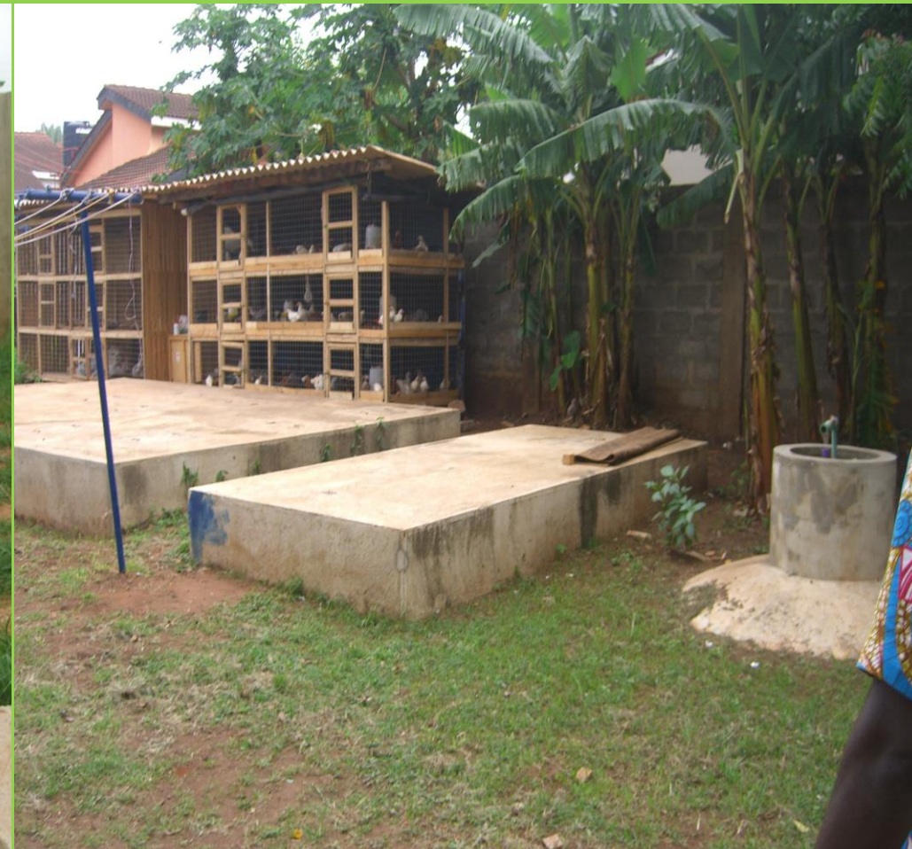
BIOGAS PLANT AT 37 MILITARY HOSPITAL TO TREAT THE FAECAL MATTER OF 160 PEOPLE
