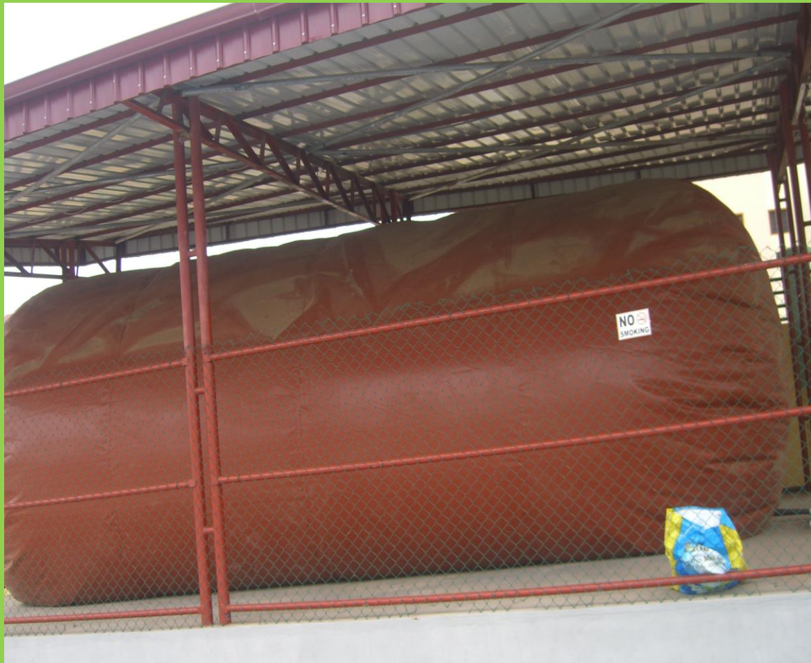
BIOGAS BALLOON FILLED WITH BIOGAS
