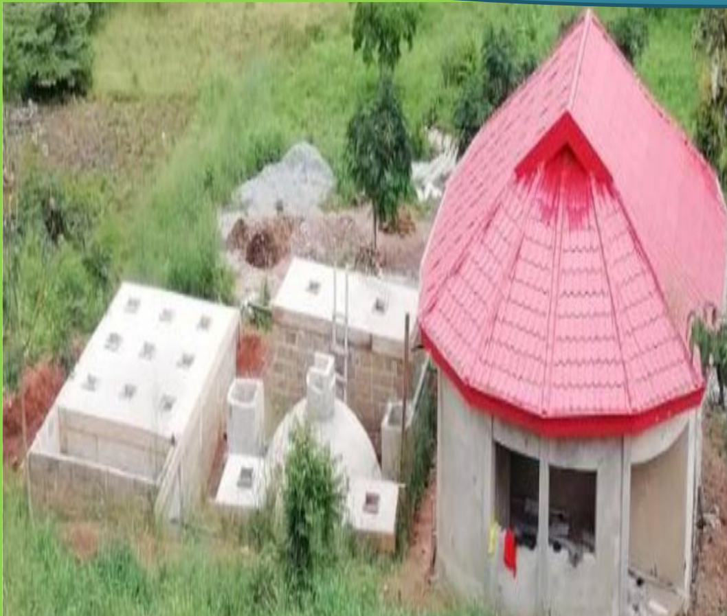
DAS FULL WASTE TREATMENT SYSTEM IN ABETIFI TO TREAT THE FOOD, TOILET AND BATHROOM WASTE OF 300 PEOPLE
