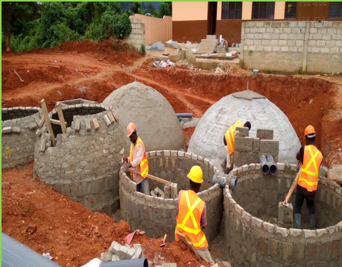
FULL WASTE TREATMENT SYSTEM AT NKAWKAW ABATTOIR PROJECT TO TREAT THE WASTE OF COWS
